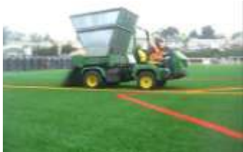
Specialist installation contractor
